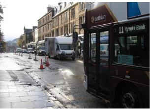
The pavement here is only 2.2m wide (ie significantly less than the SDG 'absolute minimum' of 2.5m), with a Clear Walking Zone of just 1.7m in places, and therefore the additional SfP walking lane (1.35m) is welcome.
