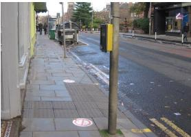
The pavement at the traffic light crossing of Morningside Road on the north side of the junction at Church Hill is only 1.9m wide, with a Clear Walking Zone of just 1.2m at the pole (right photo) – ie both substantially less than the SDG 'absolute minimum'. Being at a crossing with a long interval between the Green Man phases, this is a location where people unavoidably congregate, in addition to those passing along Morningside Road.
