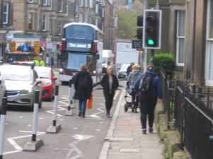
This is one of the most valuable improvements made by the SfP project along the A702 corridor. The pavement proper is only 1.39m wide (ie substantially less than the SDG 2.5m 'absolute minimum') and therefore the additional space beside a very popular pedestrian crossing is most welcome. The extra space reduces the width of the vehicle carriageway – and therefore also reduces the time taken to cross the crossing
