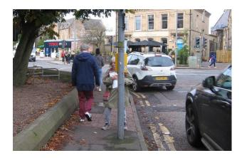
The pavement width here is only 1.7m (ie significantly less than the SDG 'absolute minimum' of 2m), and the Clear Walking Zone is just 1.1m (ie substantially less than the SDG 'absolute minimum' of 1.5m). There are long waits for the Green Man phase, during which large numbers of pedestrians can congregate in a way where it is impossible to maintain social distancing.
