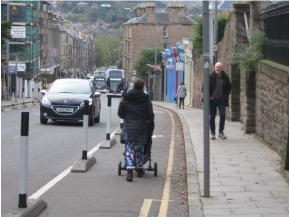
The pavement here is only 1.65m wide (ie substantially less than the SDG 'absolute minimum' of 2.5m) and the Clear Walking Zone is just 1.15m in places. (ie substantially less than the SDG 'absolute minimum' of 1.5m)
