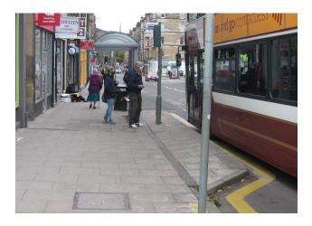
This is a good example of a bus stop build-out, allowing the pavement proper to extend to 4.4m width – one of the very few examples on the corridor where the width satisfies the SDG 'desirable minimum' of 4m or wider. The build-out also improves bus reliability, as buses do not have to wait for a gap in traffic to pull out into the main carriageway.
