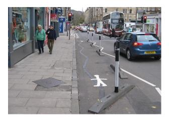
The pavement here is only 2.45m wide (ie less than the SDG 'absolute minimum' of 2.5m) and therefore the additional 1.5m SfP space is welcome. The latter also shortens the distance for pedestrians to cross the vehicle carriageway at the formal crossing in the middle distance. The angled concrete block in the foreground is not delineated by a white line, and this could represent a trip hazard.
