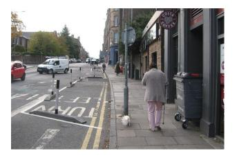
The pavement here is only 2.2m wide (ie less than the SDG 'general minimum' of 2.5m), and the Clear Walking Zone at the pole is just 1.65m. As queuing outside Luca's is common in the summer, the additional SfP space is welcome as a 'social' space and also a 'movement' space.
